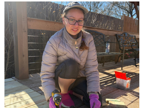
Sarah building a deck extension
